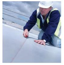
Correctly applied Sarnafil welds are stronger than the surrounding membrane. Our installer training pays particular attention to detailing around roof features.
